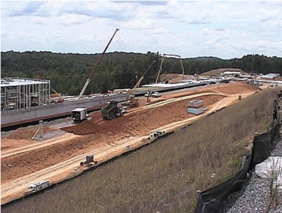
Fig. 2. Linac and helium refrigeration building.
