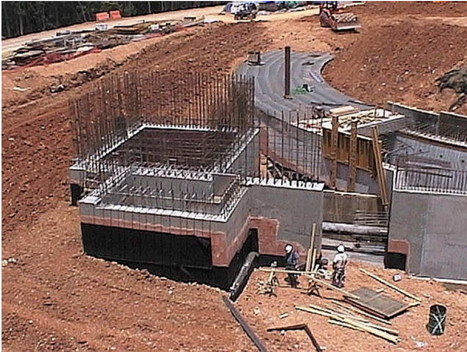
Fig. 4. Ring Injection Dump (200 kW, actively cooled). H^- that are not converted in the stripping foils to protons are accumulated here. Part of the Ring can be seen in the background.
